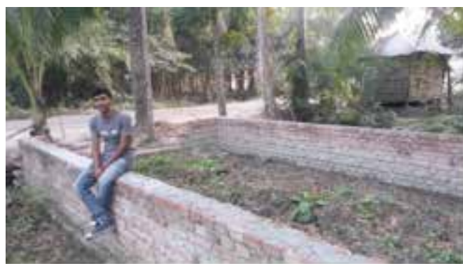
Youth club building waiting completion
